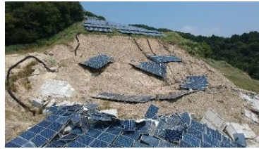
Causes a landslide
